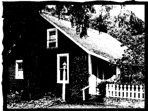
The Daley House on Moraga Blvd. was originally built as a barn in 1850.
